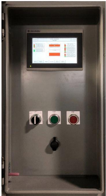
The interface includes a three-position mode switch, with start and stop buttons, that is used to select the Operating Mode.
